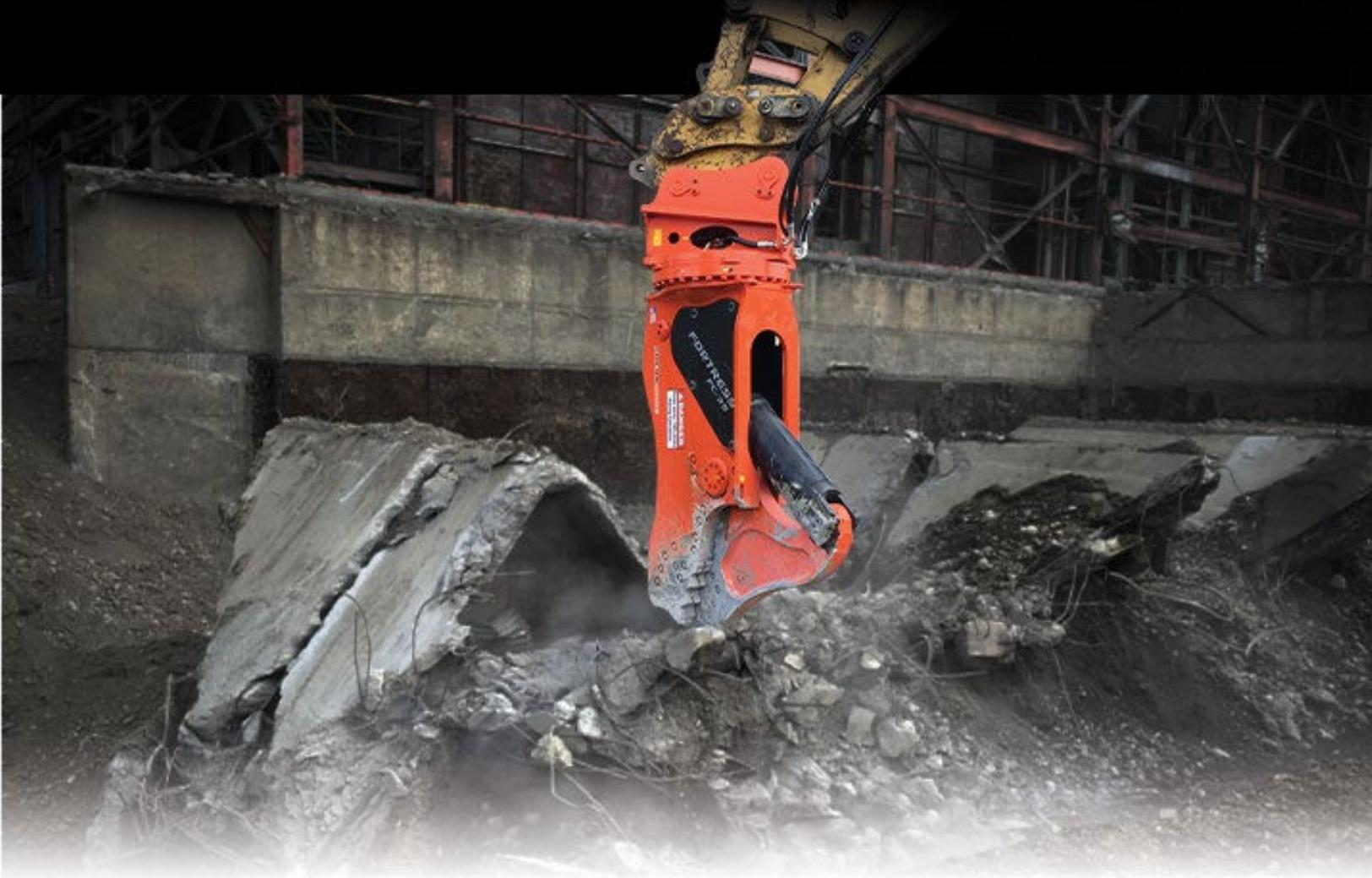
The FC can be installed on a variety of carriers; everything from smaller excavators up to massive high reach demo machines. Demolition shears are rated for up to 5500 psi.
